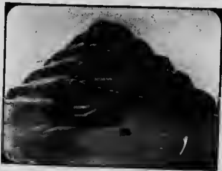
IV. The "STEP-PYRAMID" at SAKKARAH, typical of the 2nd Stage of Pyramid Building, following Medum (Front-plate "H") and resembling the Babylonian "Zigurats" outlined on Plate E. I have added the probable tier-slope-lines to indicate the easy Inclines for hauling stones up the north-shaded slope.
