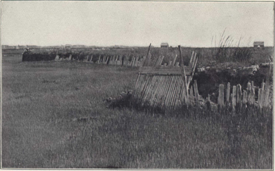
A PORTION OF THE DYKES AT GRAND PRÉ
