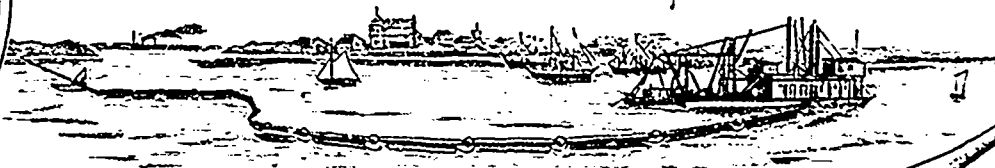
HYDRAULIC DREDGE DISCHARGING THROUGH ONE HALF MILE OF PIPE.
