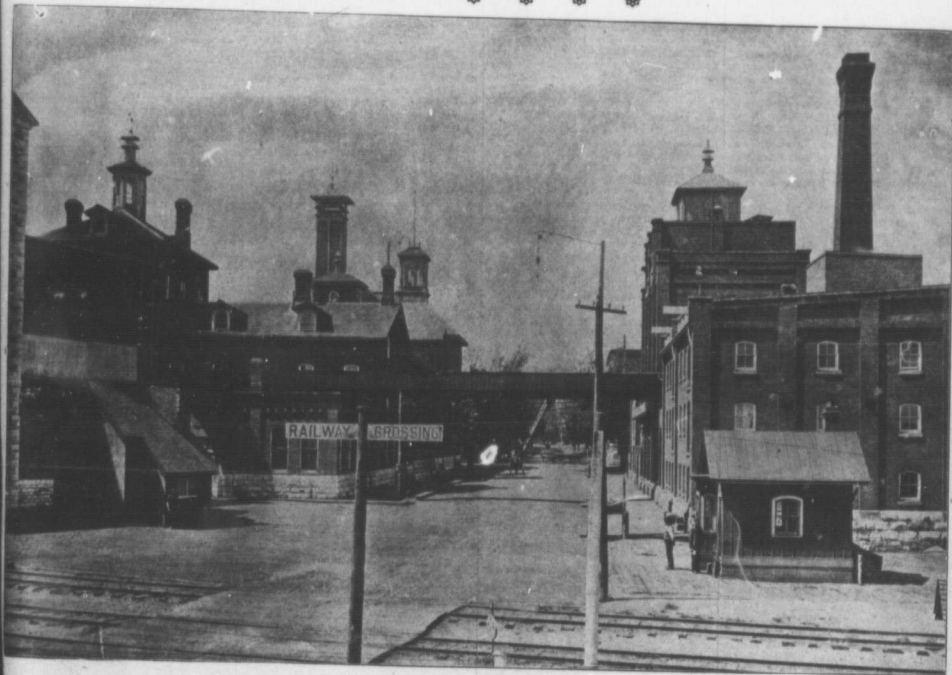
VIEW FROM THE RAILWAY LOOKING NORTH.
