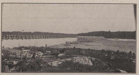
View showing River Wall and Rockfill Dam, which will divert the Flow of the Winnipeg River to the Intake Canal.
