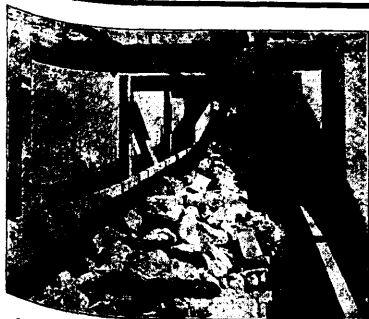
Conveyor 328 feet centers, handling 4 tons "run of mine" coal per minute.
