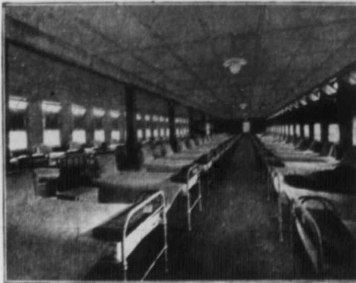
Eighty-four bed Ward at Manitoba Military Hospital. Interior finished with Gypsofibre Wall board.
