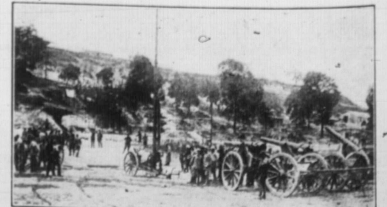
Guns of an Ally which have been taken after being turned against French. All the guns shown in this picture were originally captured by the Belgians. They were captured by the Germans in their victorious sweep through Belgium and after being repaired they were pressed into service and used in the fighting on the Somme front. The French recaptured them during the present big Allied offensive. In the centre is a giant portable captured from the Germans. This instrument is perfectly made and can be raised to a height of 20 yards. It folds up into the shape of a cannon and is drawn by horses.
