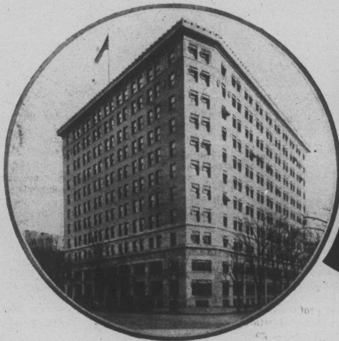
A new Government building at Washington.
