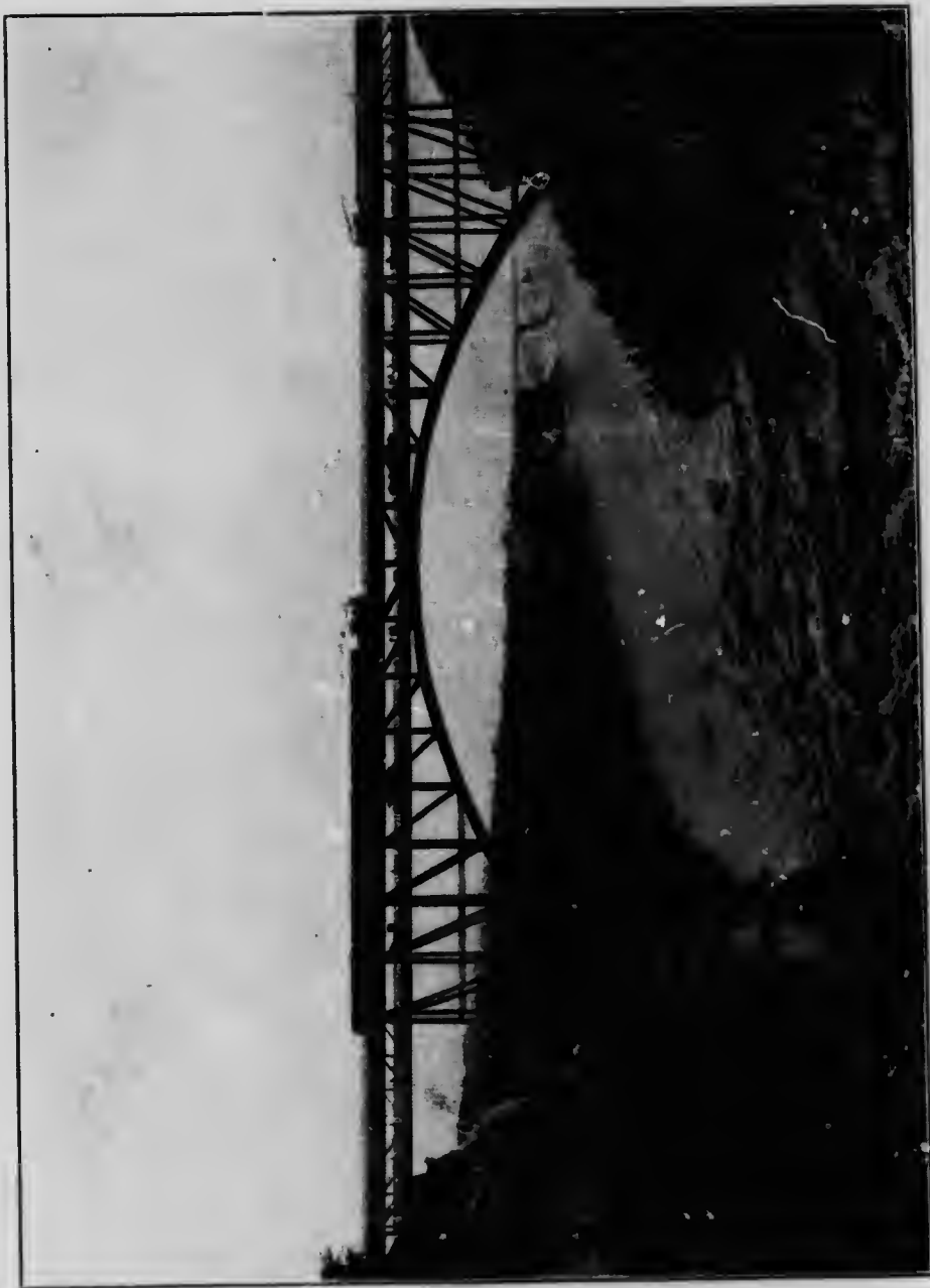
GRAND TRUNK SINGLE-ARCH DOUBLE-TRACK STEEL BRIDGE ACROSS NIAGARA'S GORGE
