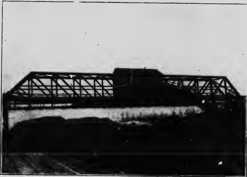
Plate XIV.—Unloading bridge, roast yard.
