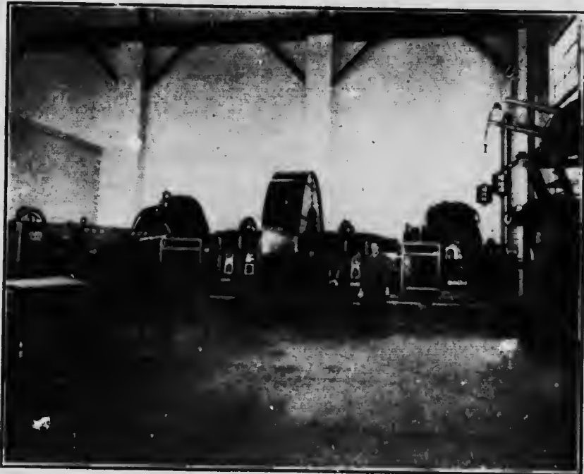
Photo by British & Colonial Press, Toronto. Plate VIII.—The motor generator set.
