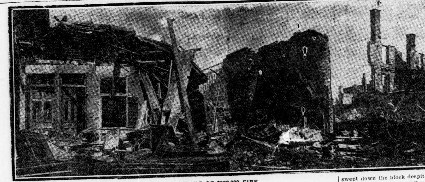
SCENE OF $500,000 FIRE. A half-million-dollar fire swept a crowded city block in Montreal Monday morning, rendering over 200 people homeless, in the most spectacular fire that Montrealers have witnessed for many years. Picture shows what is left of the Millette apartment house.
