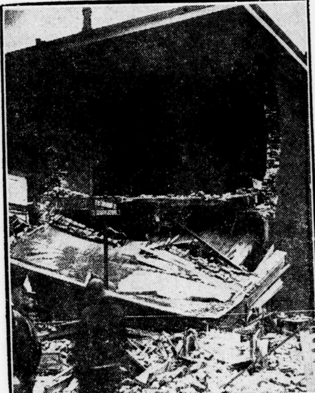
Sounds like a "whopper" to say that all this havoc was caused by a single motor truck, but it's a fact nevertheless. The heavy truck struck a supporting pillar of the building and the whole front of the structure collapsed
