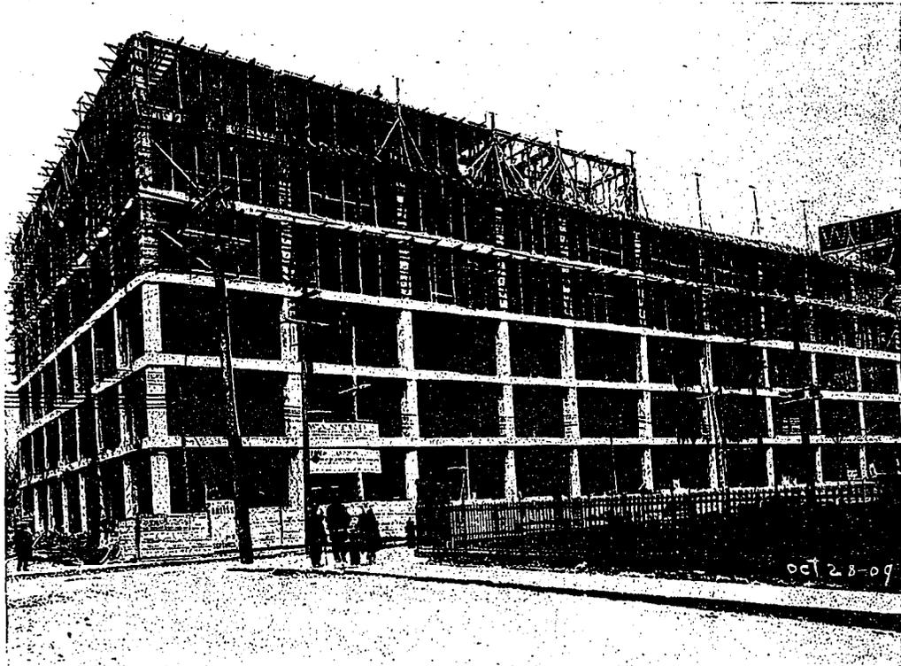
New Jacobs Building, Montreal, as it appeared on October 28th, seventy days after the foundation was completed. This view gives an excellent idea of the rapidity with which the work progressed. The time required for setting up the forms for the ground floor was ten days, and for the other floors, an average of eight days to the floor. Mitchell and Creighton, Architects.
