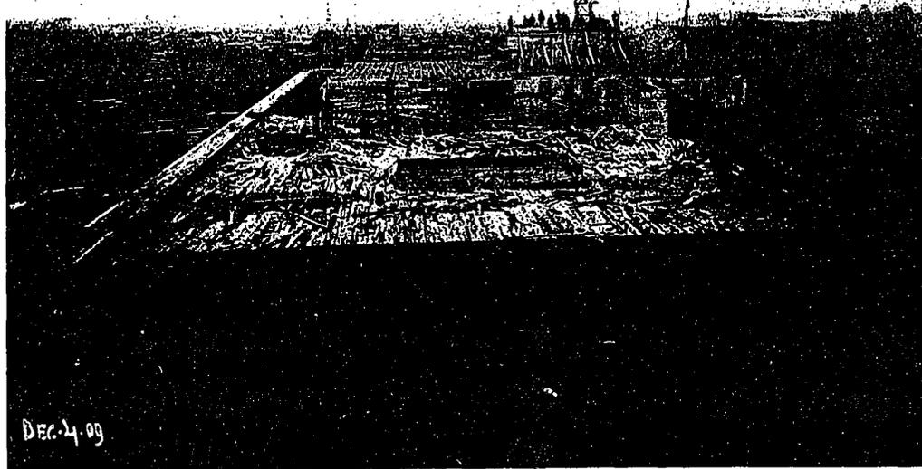
View of new Jacobs Building, Montreal, taken on December 4th, showing the building practically enclosed, and also the superstructure or seventh floor, which will eventually cover the entire area of the building and form a portion of the future extension of four floors provided for in the design and construction of the building. Mitchell and Creighton, Architects.
