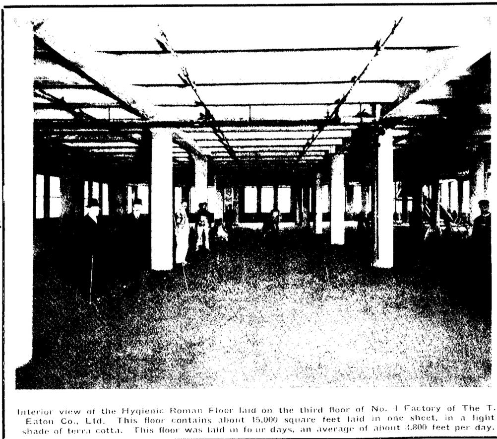
Interior view of the Hygienic Roman Floor laid on the third floor of No. 1 Factory of The T. Eaton Co., Ltd. This floor contains about 15,000 square feet laid in one sheet, in a light shade of terra cotta. This floor was laid in four days, an average of about 3,800 feet per day.
