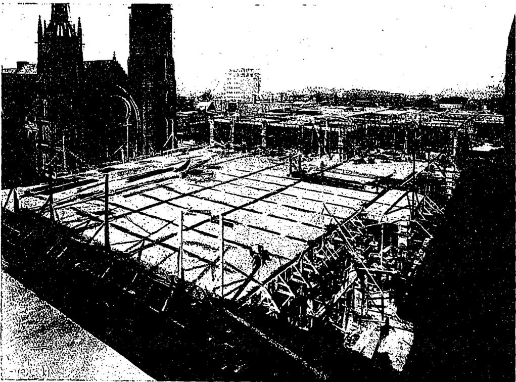
View of the new Jacobs Building, Montreal, taken on October 9th, showing the construction of superstructure. The foreground shows the finished centering ready for concreting, and the background the form work in course of erection for the next floor. The large building under course of erection in the distance, is another modern business structure which is being built according to the same system of construction. Mitchell and Creighton, Architects.
