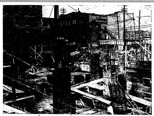
Foundation work on the new Jacobs Building, St. Catherine and St. Alexander streets, Montreal, showing the calssons and reinforcing for the concrete supporting piers. The site of the structure covers an area of 30,000 square feet and 85 piers in all were required. This view was taken on August 5th, 1909, thirteen days before the superstructure was started, and while excavation was still in progress. Mitchell and Creighton, Architects.
