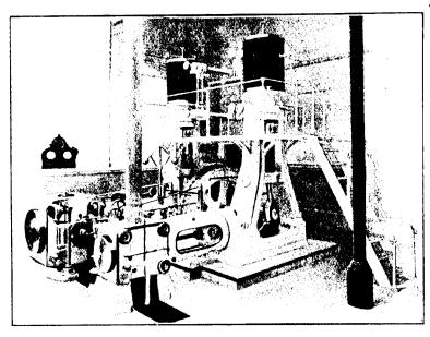
Vertical Single acting Compr ssor Driven by Compound Sweam Engine
