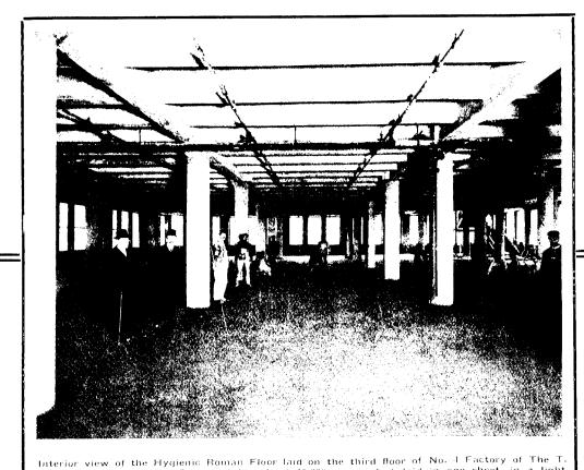
Interior view of the Hygienic Roman Floor laid on the third floor of No. 4 Factory of The T. Eaton Co., Ltd. This floor contains about 15,000 square feet laid in one sheet, in a light shade of terra cotta. This floor was laid in four days, an average of about 3,800 feet per day.
