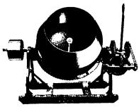
The attention of contractors is particularly called to our Open Drum Batch Mixers. The only Mixer on the market which mixes the material in sight of the operator, permitting proper gauge of the material and moisture desired, and examination as to when batch is ready to dump, it is also cleanable to an extent which entirely eliminates the caking of concrete, imparting to the machine long lasting qualities.
