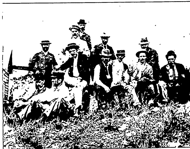
GROUP AT THE JOHNSON'S MINE.
