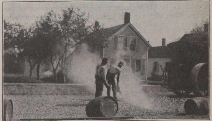
Wrong Way to Use Pouring Cans
