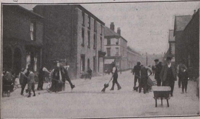
Construction of Pitchmac Pavement, Liverpool
