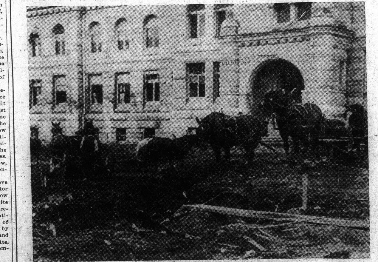
Clearing ground for new Parliamentary Annex
