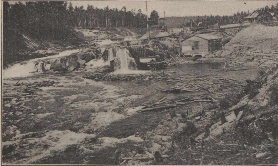
Cobalt Hydraulic Power Company. Looking Down Montreal River from point near Intake—Head-house of Intake in Distance.
