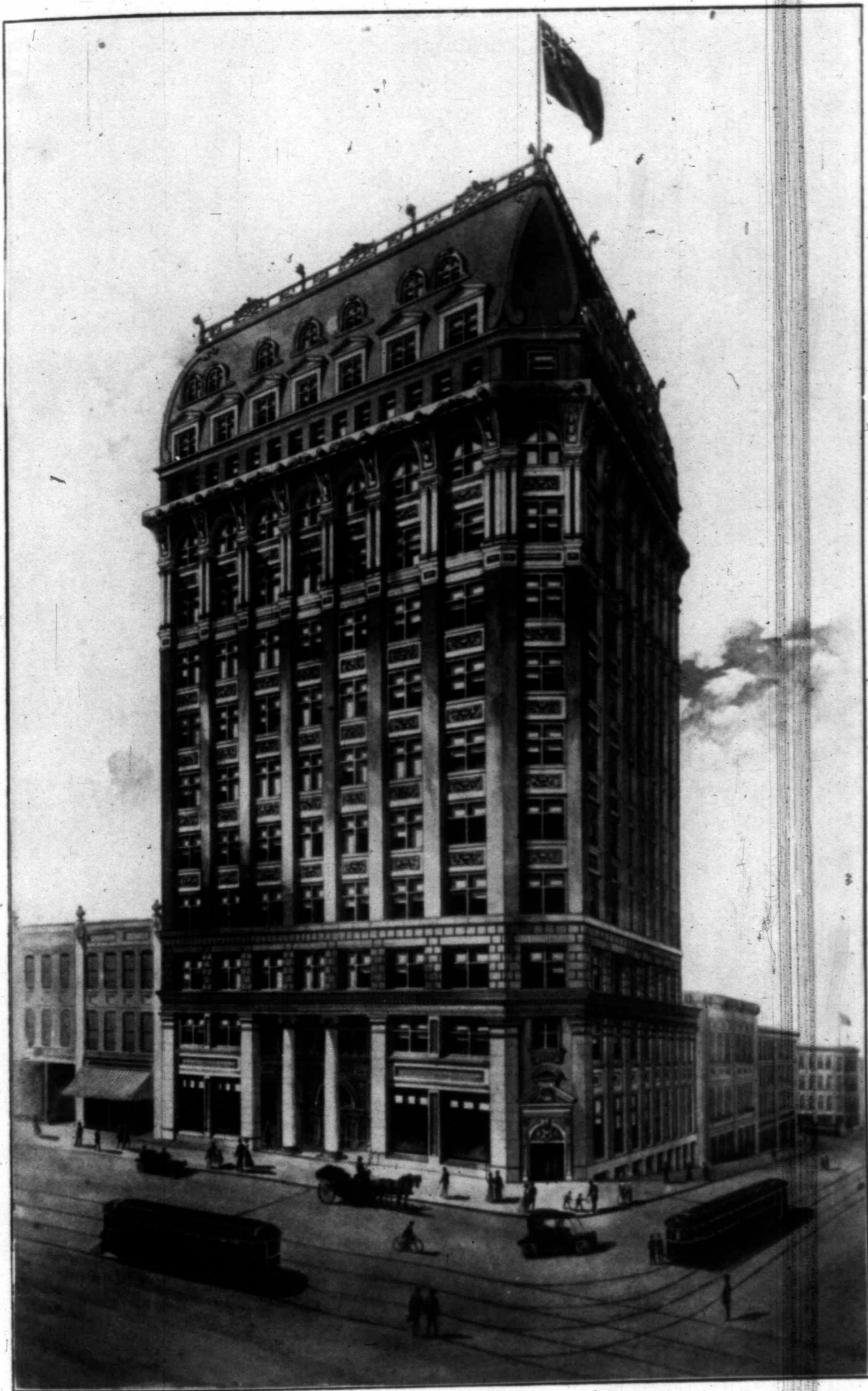
THE NEW OFFICE BUILDING OF THE DOMINION TRUST COMPANY, LIMITED. NOW BEING ERECTED AT THE CORNER OF HASTINGS AND CAMBIE STREETS, VANCOUVER, B.C. THIS SPLENDID BUILDING IS TYPICAL OF THE REMARKABLE DEVELOPMENTS OF THE COMPANY WHICH ERECTED IT, AND WHICH IS ALREADY WELL-KNOWN AS ONE OF THE LEADING TRUST COMPANIES OF WESTERN CANADA. ITS LOCATION IN THE HEART OF THE FINANCIAL DISTRICT IN VANCOUVER MAKES IT A MOST DESIRABLE HEADQUARTERS FOR ALL INSURANCE AND OTHER FINANCIAL COMPANIES DESIRING A BRANCH OFFICE IN THAT CITY.
