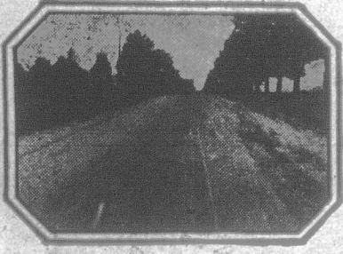
After same road was built with Tarvia Filled Macadam
