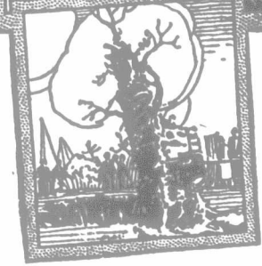
80 stumps in 100 minutes. Record made by Kirstin Horse Power Puller under official watch test at the Land Clearing Demonstration of the University of Wisconsin.
