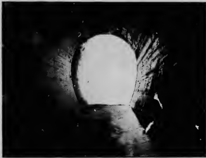
PORTAL OF TAILRACE TUNNEL, WHICH DISCHARGES DIRECTLY BEHIND THE CENTRE OF THE HORSE SHOE FALLS, ABOUT 150 FEET BELOW THE BRINK, AND ABOUT 8 FEET ABOVE HIGH WATER OF THE LOWER RIVER.
