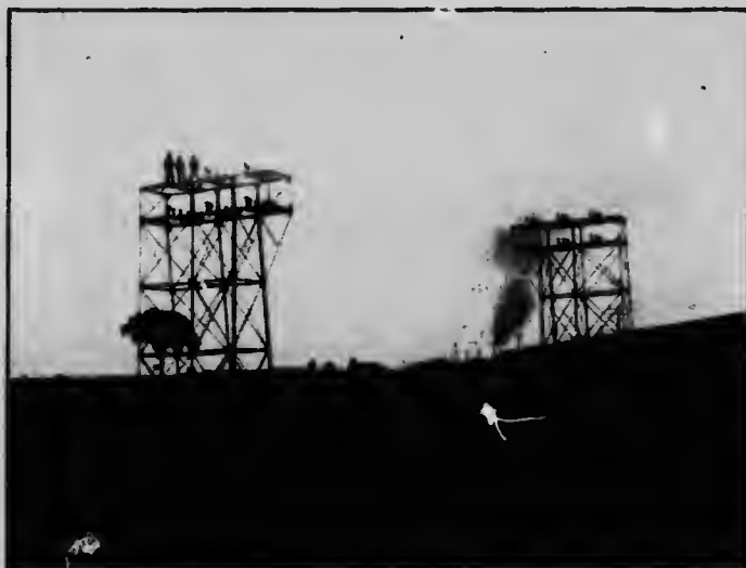
TRANSMISSION LINE, CONSTRUCTION MAIN LINE, NEAR BRONTE.
