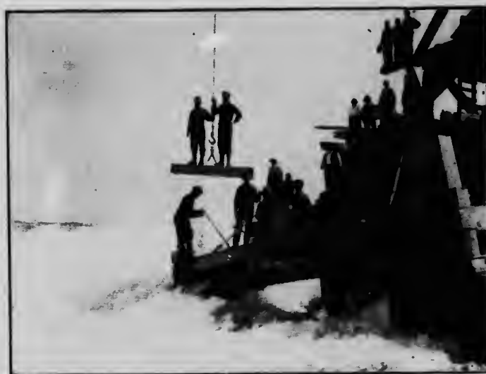
COFFERDAM CONSTRUCTION IN CASCADE ABOVE FALLS. WATER AT THIS POINT ABOUT 26 FEET DEEP, AND VELOCITY OF 22 FEET PER SECOND.
