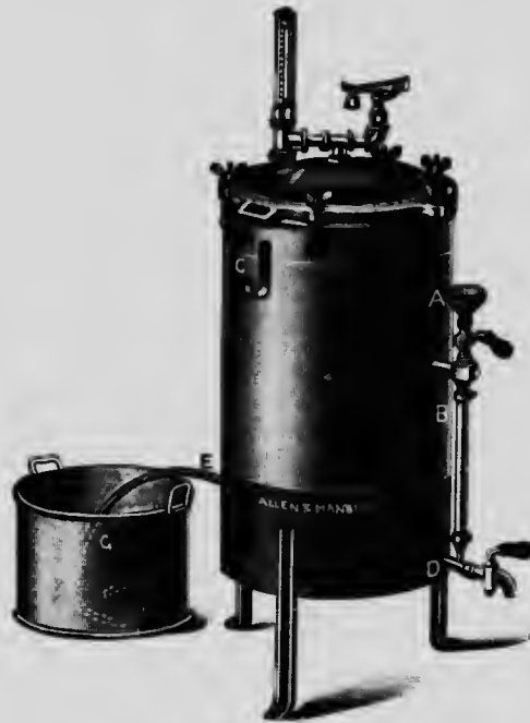
Fig. 288.—High pressure steam sterilizer.
