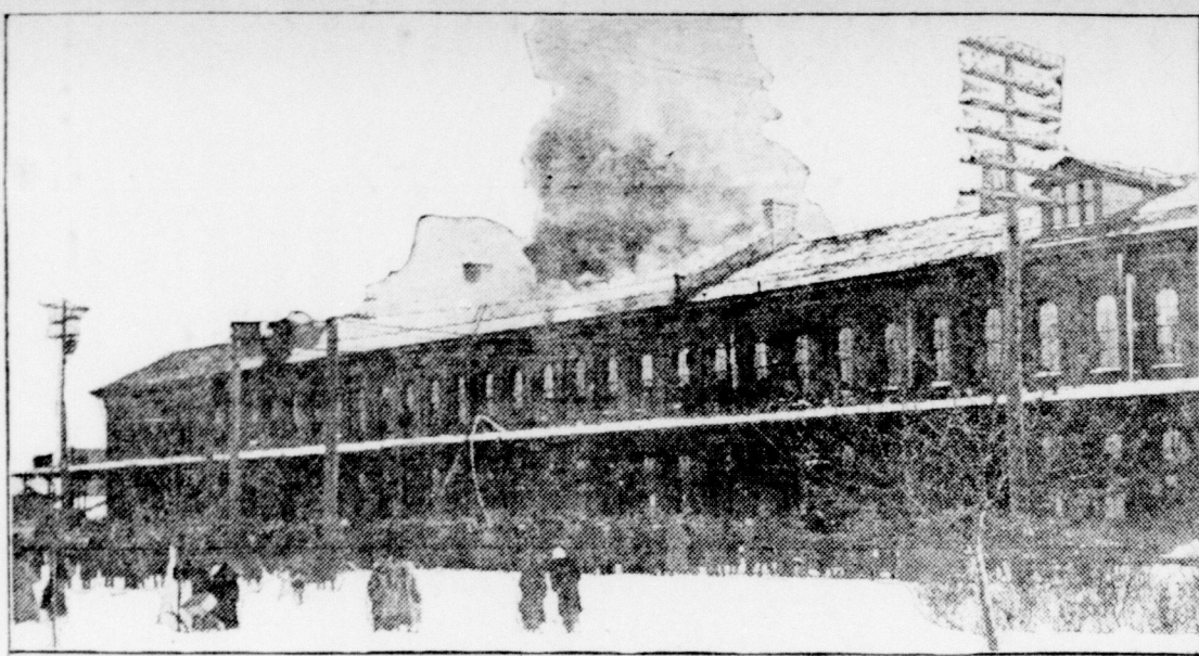
M. C. R. DEPOT AT ST. THOMAS IN FLAMES. Railway since that company took over the Canada Southern some years ago.
