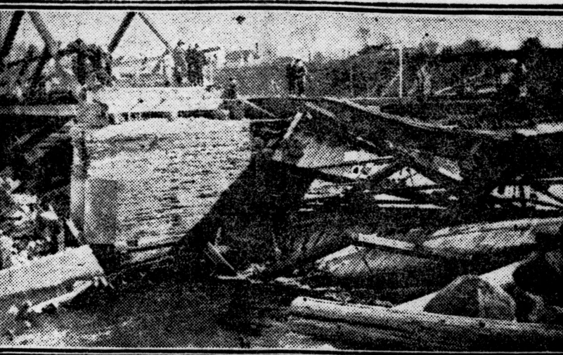
This photograph was taken shortly after the structure gave way. The collapse was due to weakening of abutments from spring freshets. It was built sixteen years ago.
