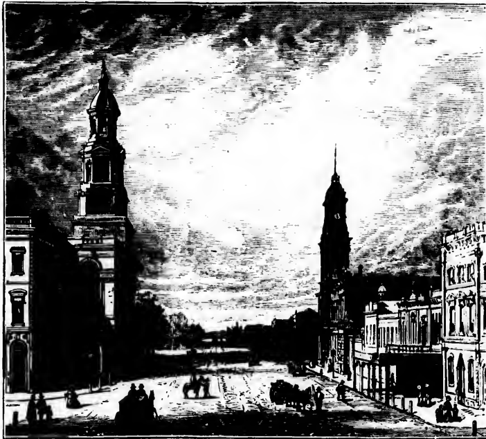
POST-OFFICE AND TOWN HALL, ADELAIDE.
