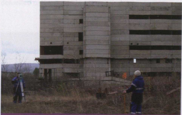
Canada's contribution to the US-led construction of an alternative energy source will enable Russia to shut down its last weapons-grade plutonium producing reactor, located in Zheleznogorsk
