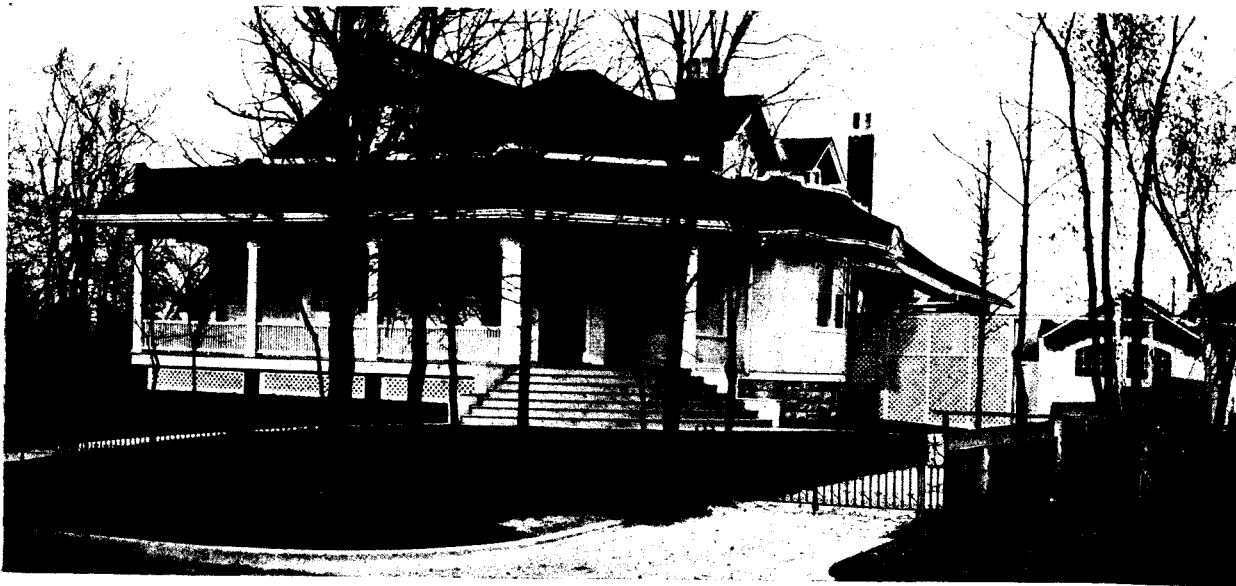
Residence of A. W. Chapman, Armstrong's Point, Winnipeg, Man. William Fingland, Architect. Randall & Bell, Plumbers. Equipped with Alexandra Ware.
