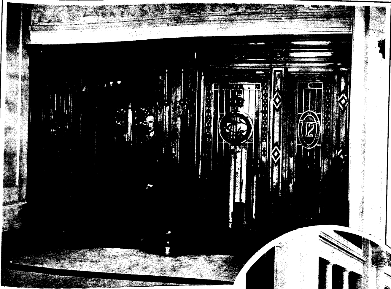
Otis Electric Passenger Elevators Installed in Chateau Laurier.
