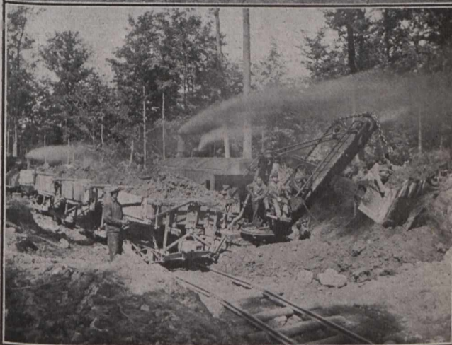
Earth Dam Construction at Eugenia Falls, Ont., Showing (1) Method of Construction; (2) Method of Excavating for Puddle Core, and (3) Transportation of Excavation from Canal.
