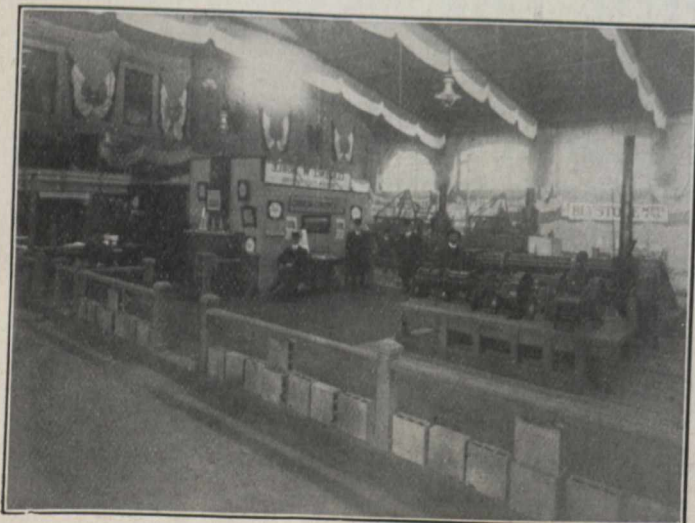
MINIATURE CEMENT MILL. Instructive Exhibit of Canada Cement Co.
