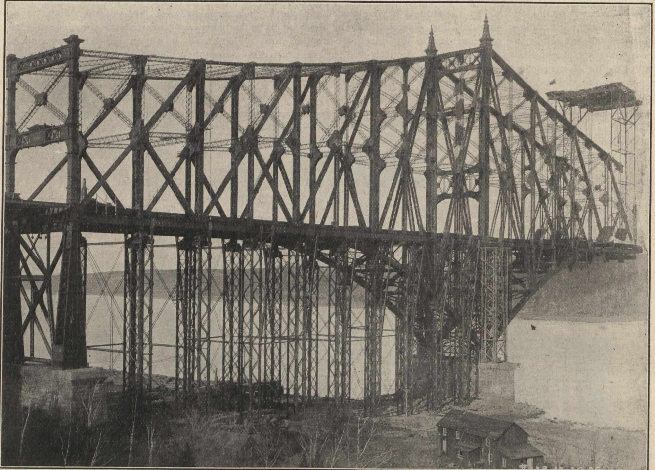
View of South Anchor and Cantilever Arm Under Construction.
