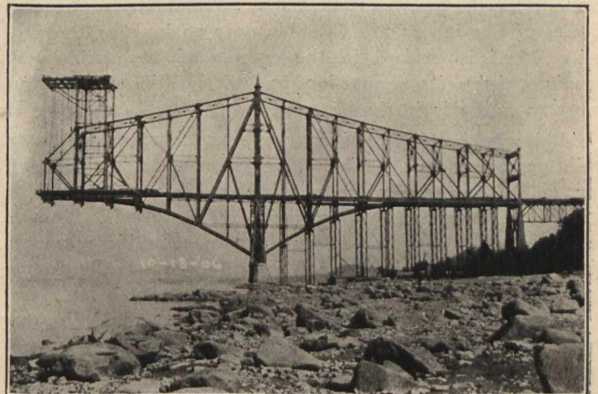
Quebec Bridge.—South Cantilever Arm.
