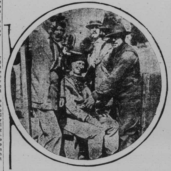
"GETTING THE LOWDOWN" On the new water system pipe being installed on the bottom of Burrard Inlet. L. D. Taylor, Vancouver's versatile mayor, recently descended in a diver's uniform.
