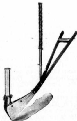
Fig. 6. Shoe of Cockshutt Hoe Drill.
