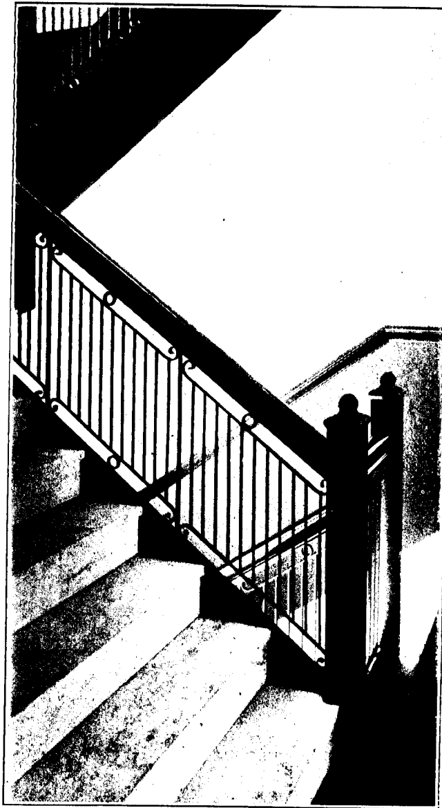
Stair railing installed by us in Y. W. C. A., Hamilton
