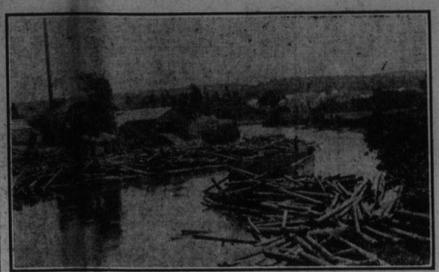
View from Apohaqui bridge showing twisted mass of logs hurled aside by the big cloudburst. Note the heavy pier which was moved and pierced by logs driven by the force of the water, and the ruined runway leading into the Jones Bros. mill.
