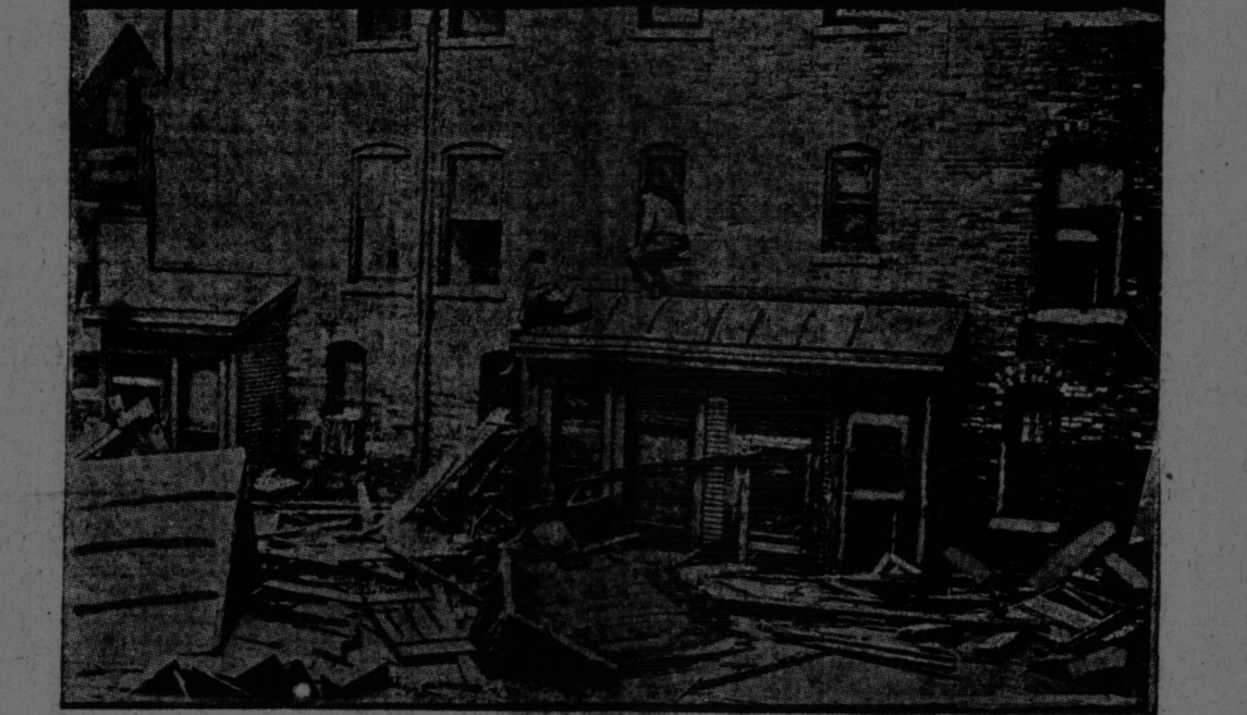
People escaping from a house in Columbus, Ohio, after the flood had somewhat subsided. Their stairs had been washed away.
