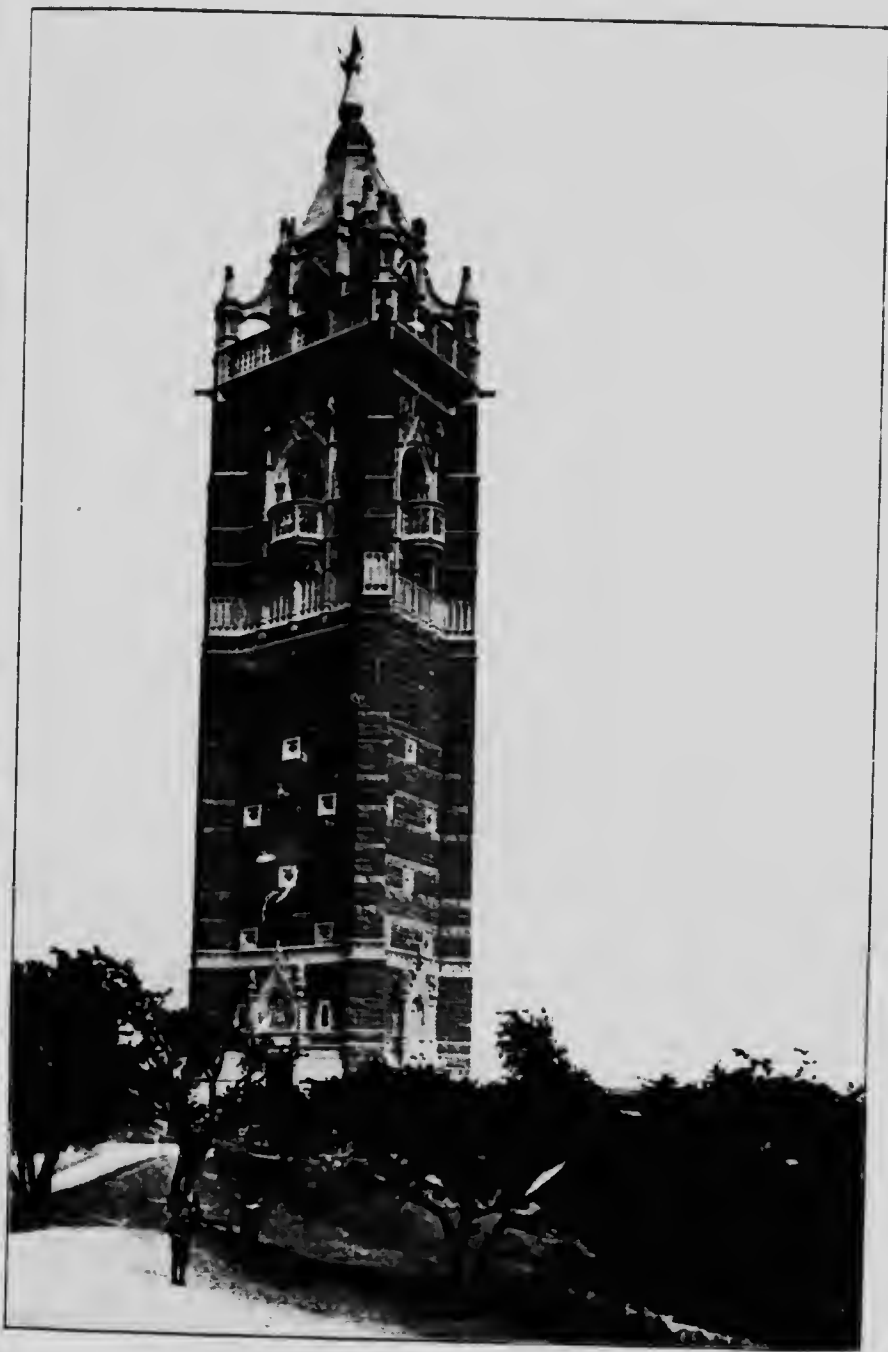
The Cabot Tower at Bristol
