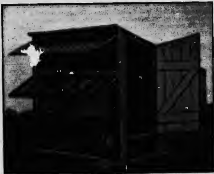
A good type of colony house. Measurements, 6 feet long, 8 feet deep, 6 feet 6 inches in front, 4 feet 6 inches rear. Colony houses can be hauled to any part of the ranch, thus giving young or old stock opportunity to range on clean soil. Can be used as cockerel, pullet, or breeding houses after chickens are matured. The top shutter or board window makes a splendid hood or rain-shield and can be changed to a muslin-curtain screen if desired.
