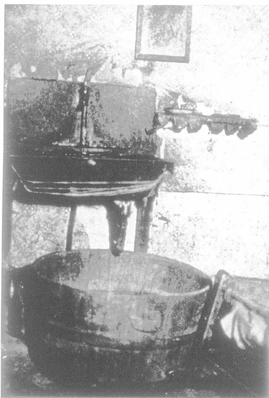
View of Plumbing in the living room of a House.
