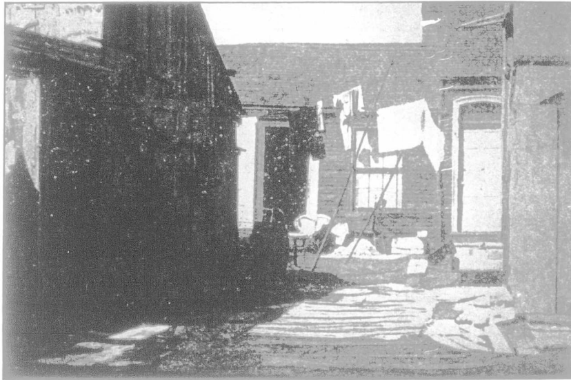
Corner of a Courtyard in which over 40 People Dwell
