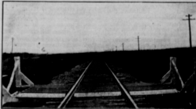
This Photo shows the new cattle guard invented by Mr. Robert B. Walker of Strathcona, Alta. The cow that tries to cross this gets a sharp crack on the shin.
