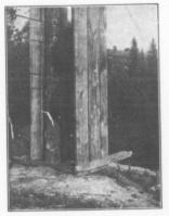
Support for the Power Cables power from Mr. Tamblyn's turbine is carried to barn by a cable as seen. This illustration shows the cables are supported and the direction changed at the brow of the hill.
