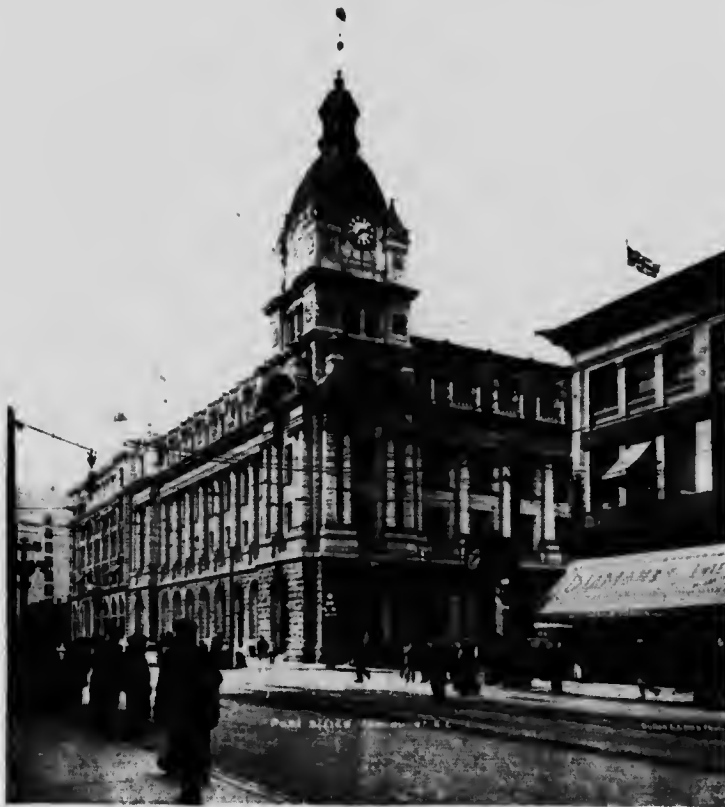
Post Office, Vancouver, B. C.
