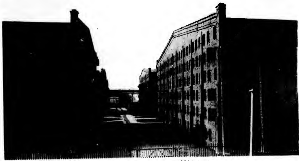
RACK WAREHOUSES, CONTAINING 50,000 BARRELS.
