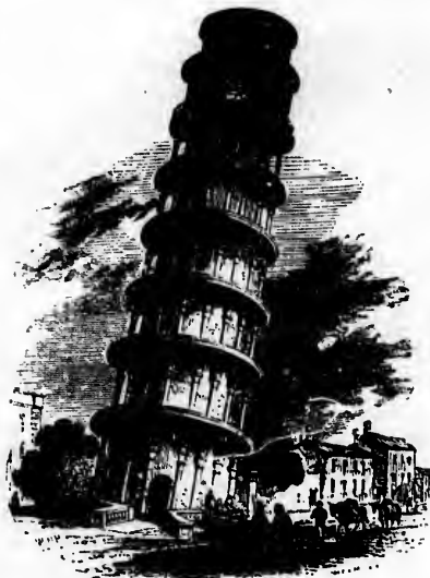
LEANING TOWER OF PISA.
