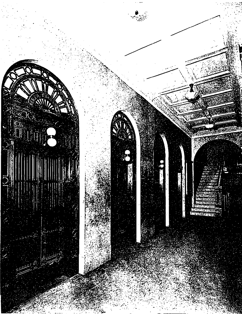
ELEVATOR HALL ON MAIN FLOOR.
