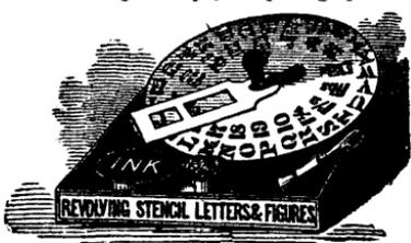
Revolving Stencils will be found useful for marking boxes, signs, etc., size of
