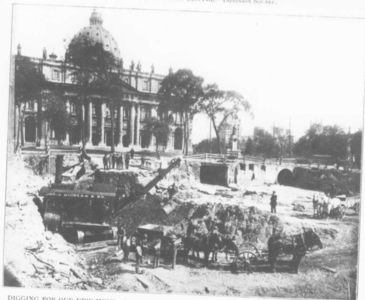
DIGGING FOR OUR NEW HOME.—EXCAVATION WORK FOR FOUNDATIONS OF NEW SUN LIFE OF CANADA BUILDING. Site is marked by X in upper picture.
