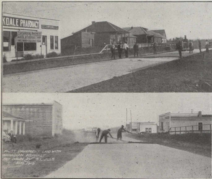
Laying the First Pavement With Canadian Asphalt, Edmonton, August, 1915.
