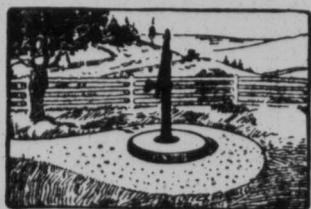
SHOWING CONCRETE WELL CURB AND PLATFORM.
