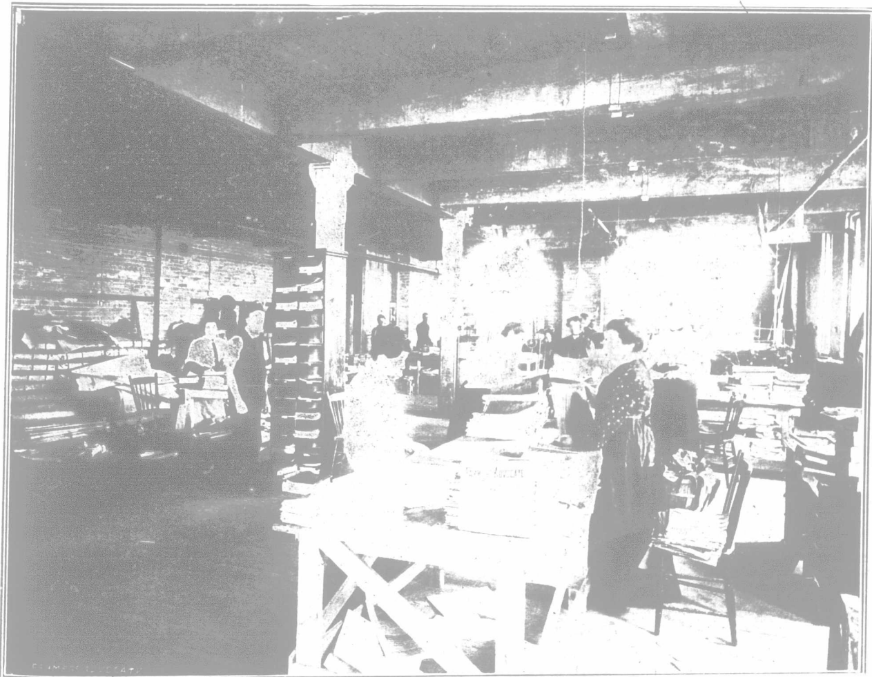
A SECTION IN THE MAILING ROOM (Fourth Floor).
